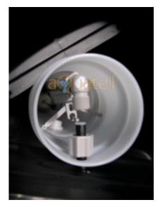
To attach the brine line to the brine tank you will first insert the tube insert into one end of the brine line. Be sure to push it all the way in. Then pass this end of the brine line through the upper hole in the brine tank and through into the brine well. Slide the hex nut onto the brine line and then insert the brine line fully into the threaded elbow of the brine float. Now tighten down the hex nut until it is snug making sure that the brine line is held firmly in place.
